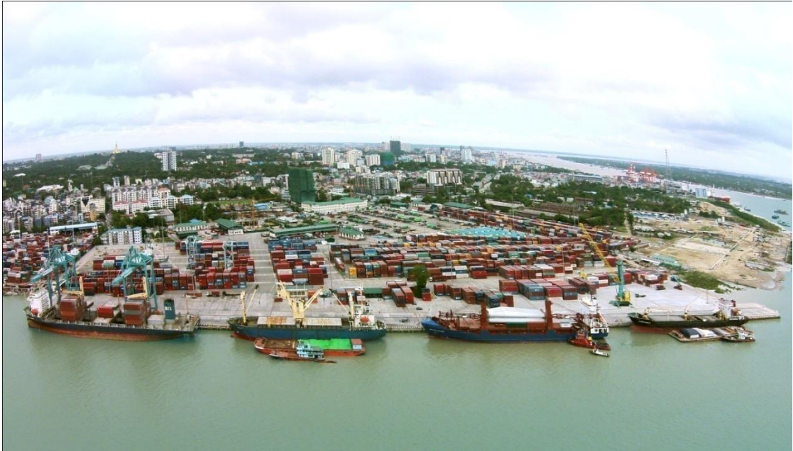
Source: Myanma Port Authority
